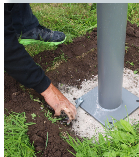
Tighten the anchors (M12 = 90 N/m and M16 = 120 N/m).
