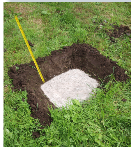
Fill with concrete leaving a depth of e.g. 25/40 cm / 10"/16" (see the following pages). Dry for approx. 6-7 days.
